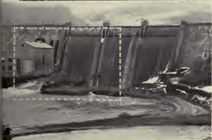
DRYING THE "TOE." —Above, close-up of the diversion facilities, showing 60-inch diameter steel pipes connected to the conduits at the face of the dam to carry discharges from sluice gates. At left, general view of the same area (outlined) before pipes were installed, showing the completed cofferdam and the diversion flume.
